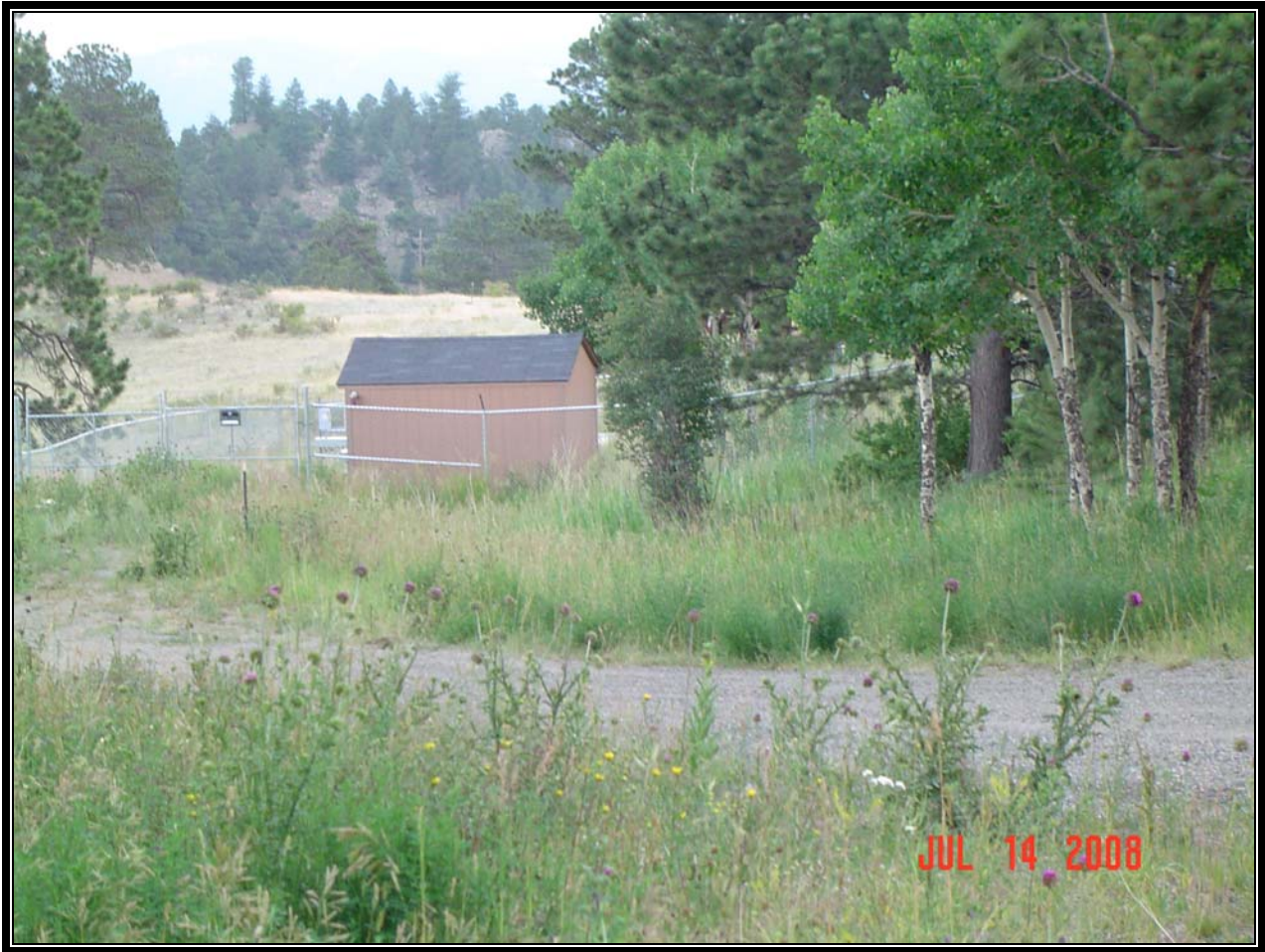
Figure 2. Equalization Basin Building
