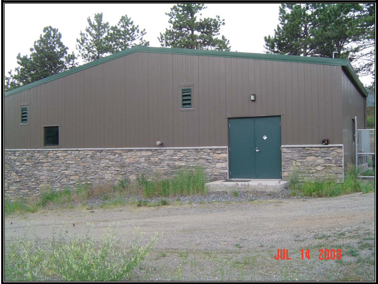
Figure 1. Treatment Facility Exterior
